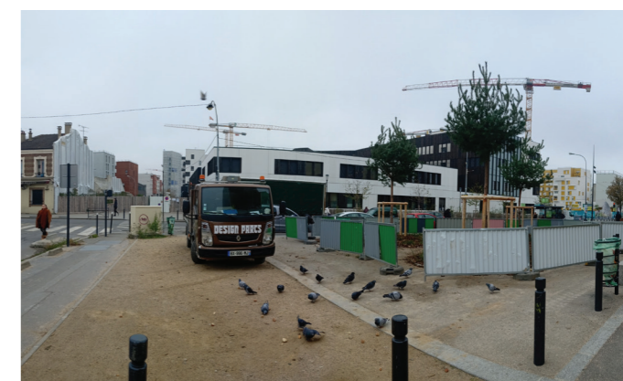
Site surveying at Plaine Commune
